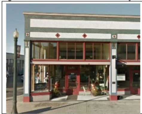
Figure 14.195-4: Prominent Main Entry
